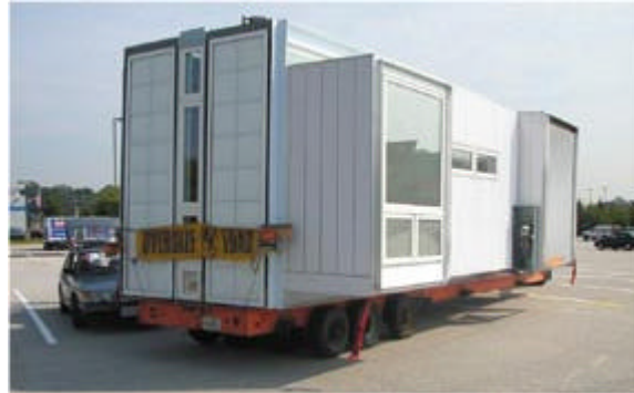
The Virginia Tech entry ready for transport to the Washington DC Capitol Mall. One of the demanding issues was to devise a structure that could be built, transported and reassembled on site efficiently. Nationwide Homes provided the transport vehicle.
