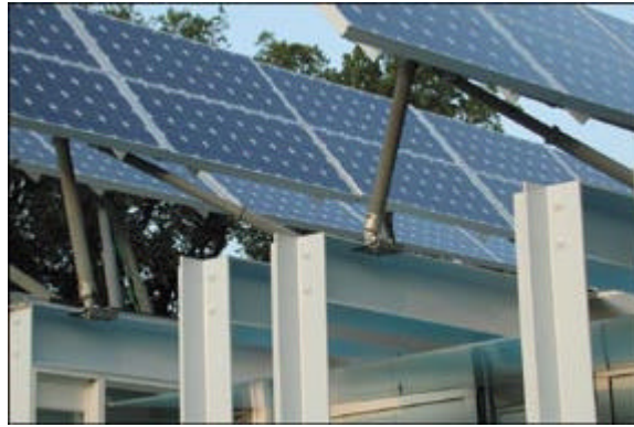
The VT solar array consisted of 80 21"X47" photovoltaic cells producing 6Kw at peak output. The panels are clamped, allowing elimination of roof penetration and resultant thermal bridging.
