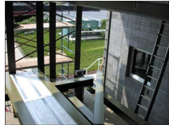
The Thermasteel SIP floor system is inserted between the fiberglass I-beams.
